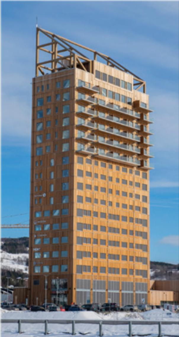
*Mjøstårnet, Norway: 18 storey post and beam structure .*
